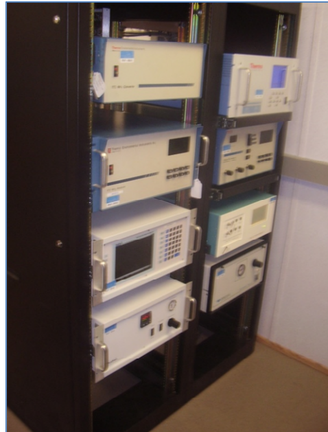
Figure 2: Typical station interior
