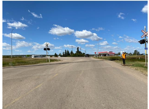
Photo 2: Looking West along 50 Avenue at railway crossing
