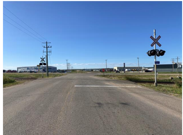
Photo 2: Looking South along Highway 831 at railway crossing
