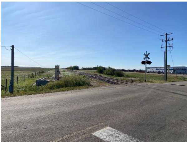
Photo 3: Looking Left from North approach
