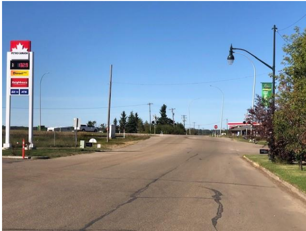
Photo 1: Looking West along 50 Avenue towards railway crossing
