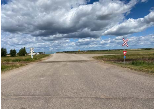
Photo 5: Looking North along Rge Rd 195 towards railway crossing
