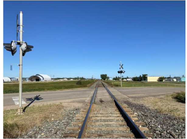
Photo 10: Looking West at Railway Crossing
