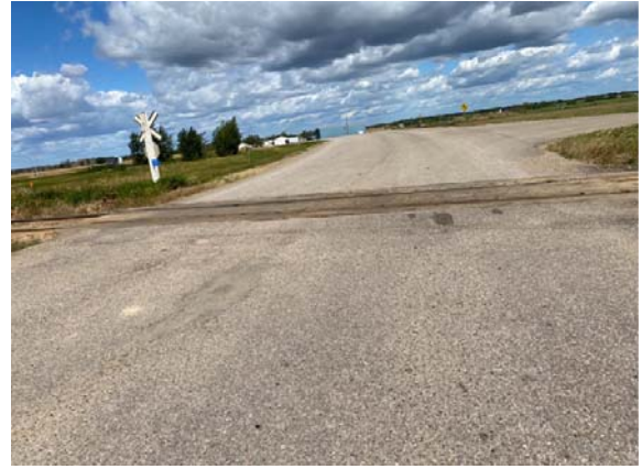
Photo 6: Looking North along Rge Rd 195 at railway crossing
