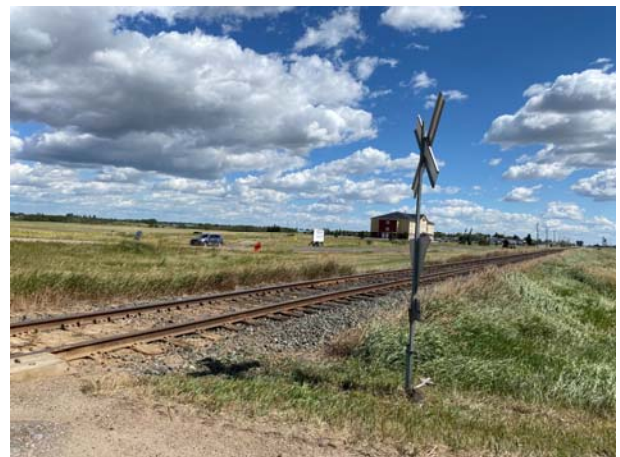
Photo 8: Looking Right from South approach
