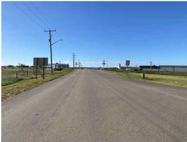
Photo 1: Looking South along Highway 831 towards railway crossing
