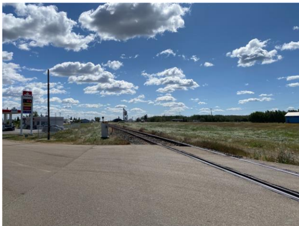
Photo 3: Looking Left from East approach
