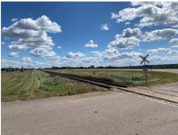
Photo 3: Looking Left from North approach
