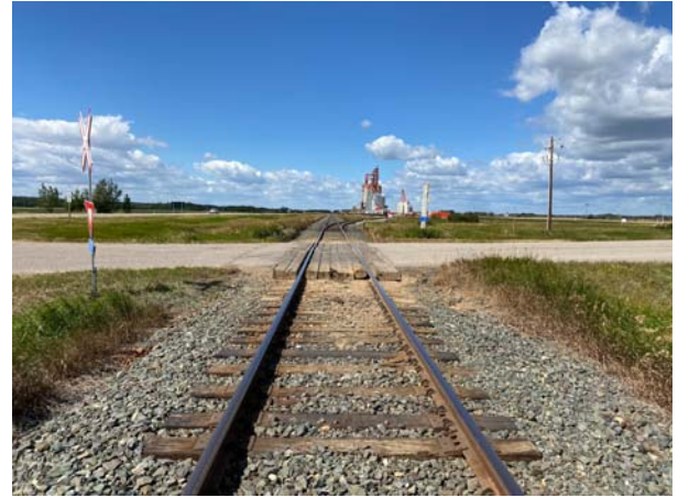
Photo 10: Looking West at Railway Crossing
