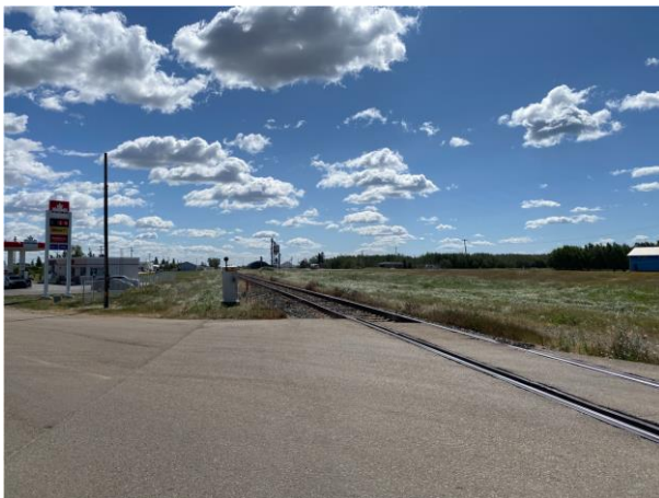
Photo 3: Looking Left from East approach
