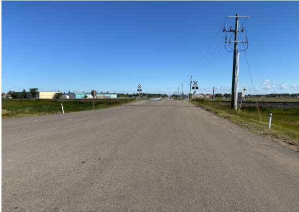
Photo 5: Looking North along Highway 831 towards railway crossing
