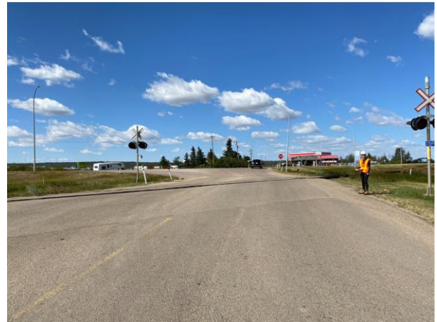
Photo 2: Looking West along 50 Avenue at railway crossing
