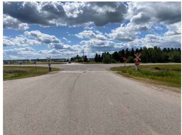
Photo 2: Looking South along Rge Rd 195 at railway crossing
