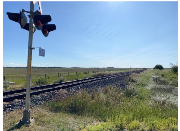
Photo 8: Looking Right from South approach
